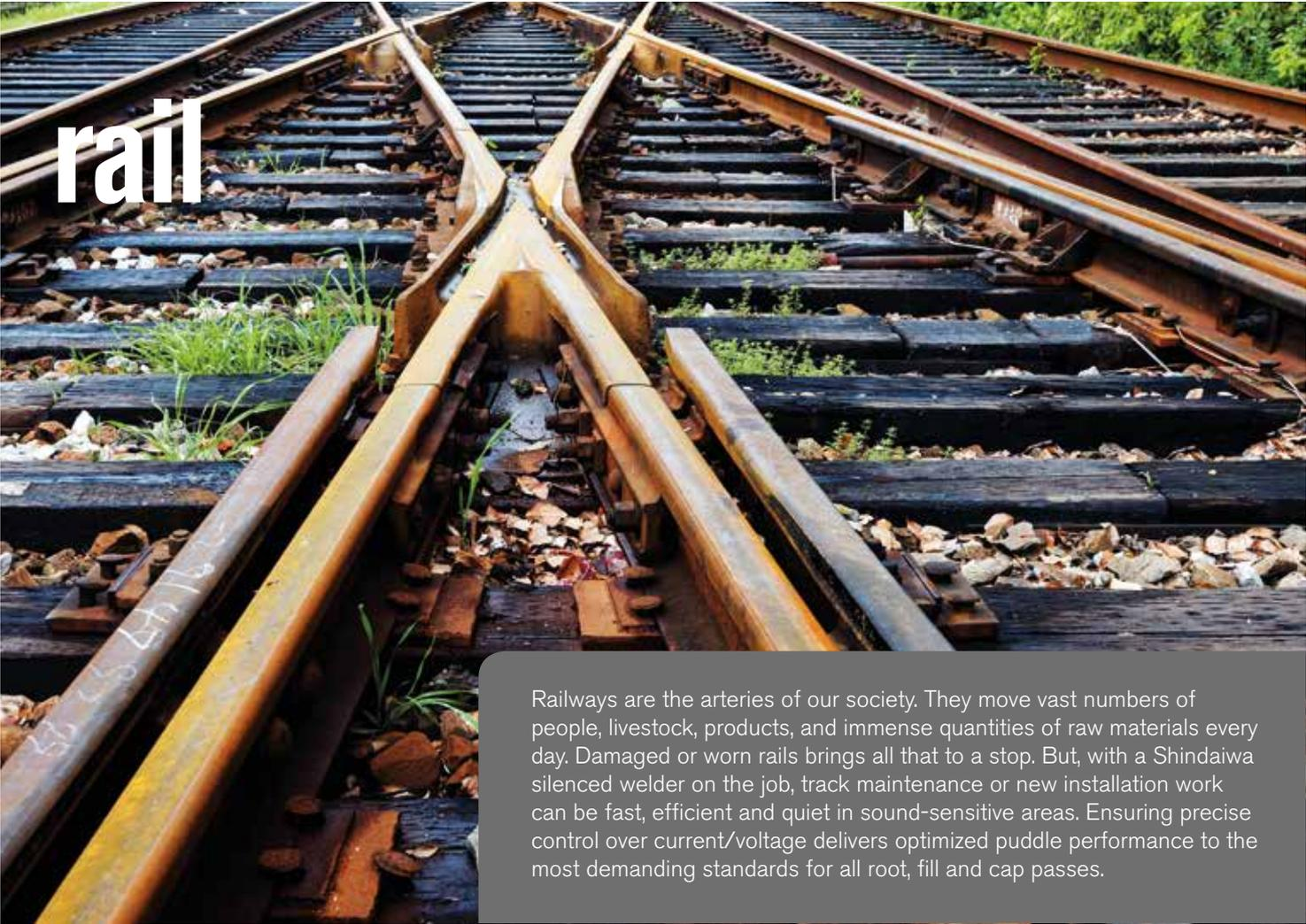
A photograph of railroad tracks receding into the distance, with a central switch or crossing. The tracks are made of steel rails on wooden ties, set on a bed of gravel. The perspective is from a low angle, looking down the tracks.
